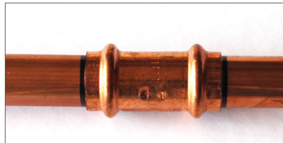
Figure 11.14. Fitting prepared for pressing
