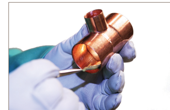
Figure 7.10. Fluxing: Fitting
