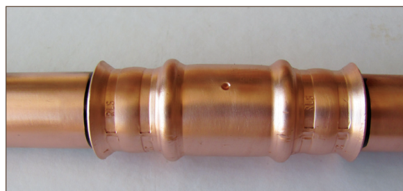
Figure 11.19. Completed joint with insertion marks visible
