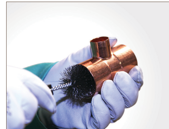
Figure 7.8. Cleaning: Fitting Brush
