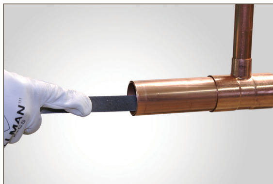
Figure 7.3. Reaming: File
