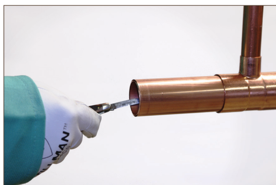
Figure 7.4. Reaming: Pocket Knife
