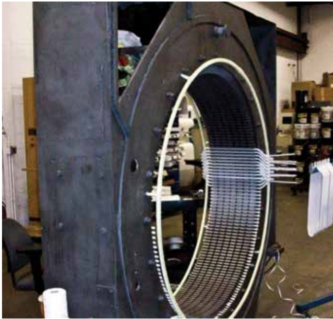
500 Horsepower motor undergoing new copper coil insertion (photo courtesy of EECO)
