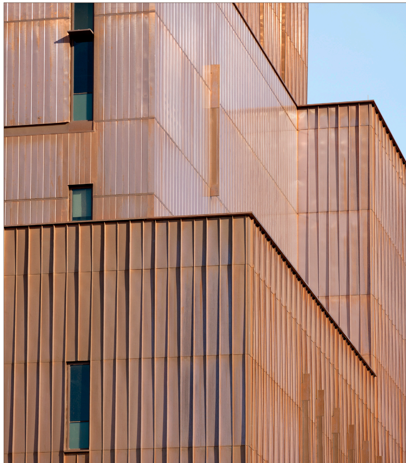
Maricopa County Downtown Court Tower, Photo Credit: Bill Timmerman
