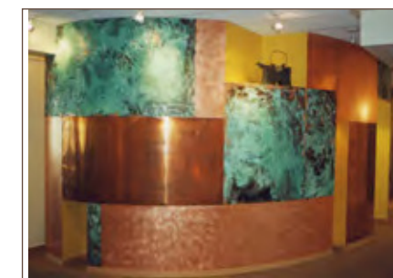
Figure 3A. This lobby in Anchorage, Alaska, artfully displays panels of copper alloys using a variety of colorful chemical and mechanical finishes.
