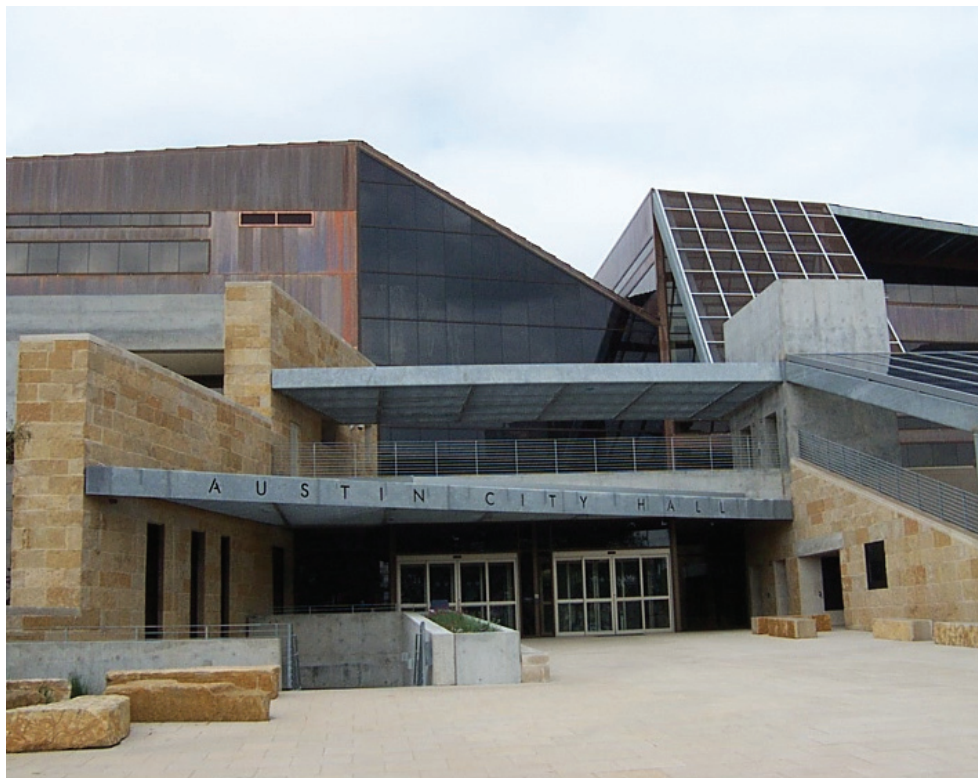
Exterior and interior uses of copper helped Austin City Hall earn USGBC's Gold LEED certification.
