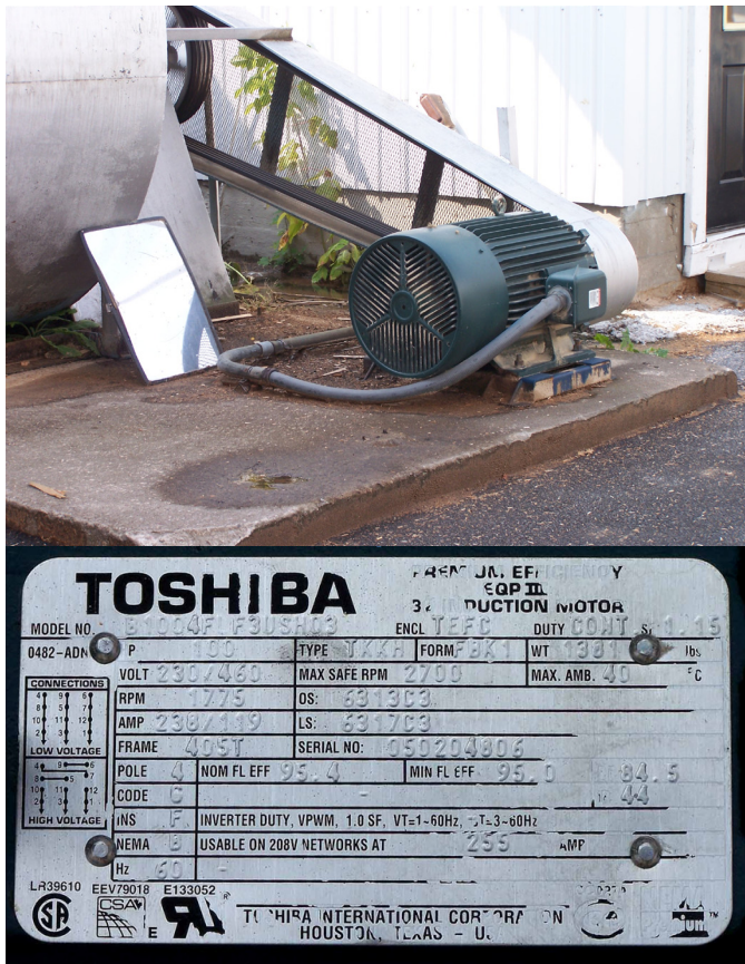
Figure 3. A NEMA Premium-rated 100-hp Toshiba EQP III now powers the large blower (top) at the plant's baghouse. The new motor operates with 95.4% efficiency (dataplate, bottom), saving the company $1880 annually in energy costs compared with the standard-efficiency motor it replaced. It paid for itself in only 2.43 years.
