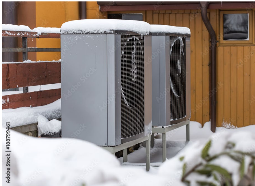
Figure 6 – Even at temperatures before freezing, today’s cold climate air source heat pumps (CC-ASHPs) deliver heating more efficiently than burning fossil-fuels or electrical resistance heating.
