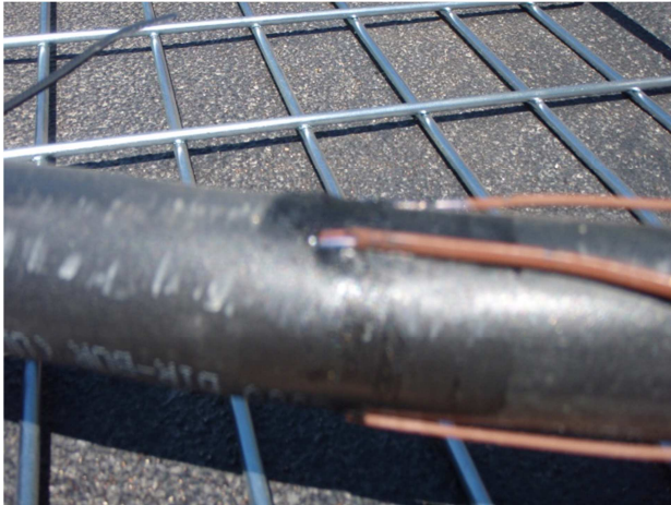
Fig. 4 – Thermocouples Installed on Conductors
