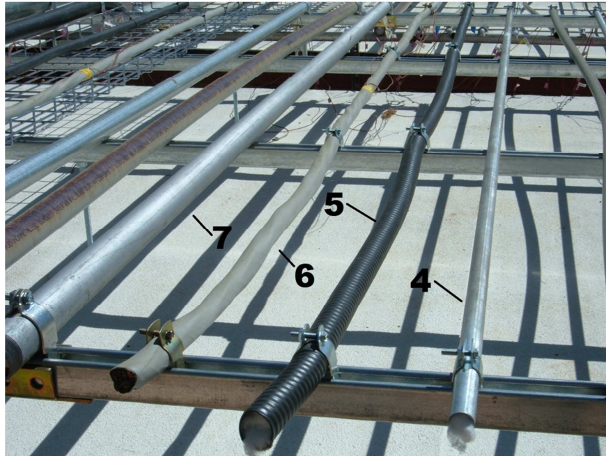
Fig. A2 – 3/4 EMT (4), No. 1/0 MC (5), No. 1/0 SE (6), 1-1/2 RMC (7)
